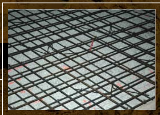
Rebar mat in concrete slab
